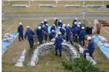
Protection of bank using plastic sheets
