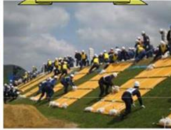
Protection of bank using plastic sheets
