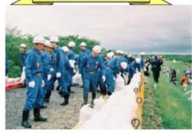
Deployment of sandbags
