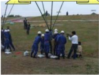
Ground crack repair by trivet-shaped binding of bamboo booms with sandbag
